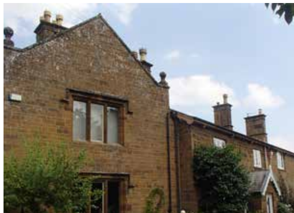
Two to three storey buildings, Adderbury
