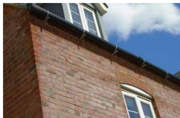
Guttering, South West Bicester
