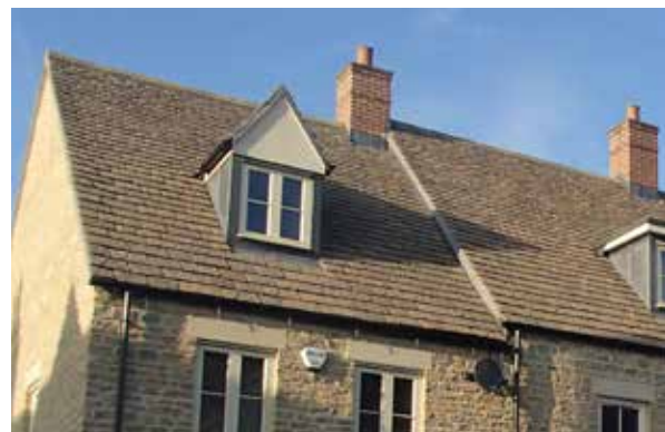
Good examples of modern dormer windows, pitched roofs, slate tiles and brick chimneys, Woodstock
