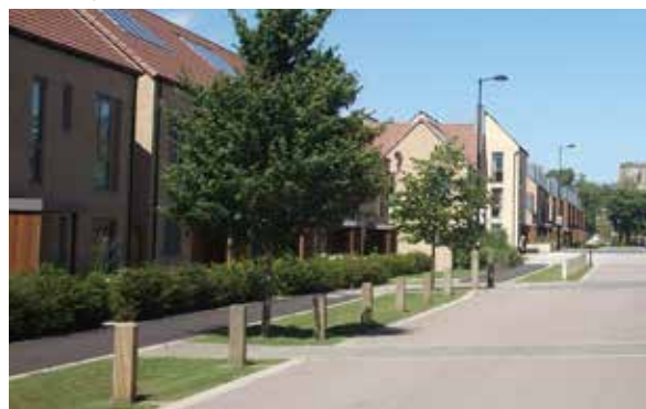
Incorporating SuDS along kerbside, Trumpington Meadows, Cambridge
